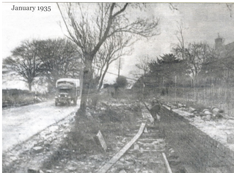
RICHARD JEFFERIES' WALL – A photograph of the work in progress on the setting back of the wall at Richard Jefferies' house at Coate, Swindon. The beginning of the new wall is seen on the right; its original position is marked by the line of trees, which were inside the fence. Its removal is due to a road widening scheme at this point, sentiment having had to give way to safety.
