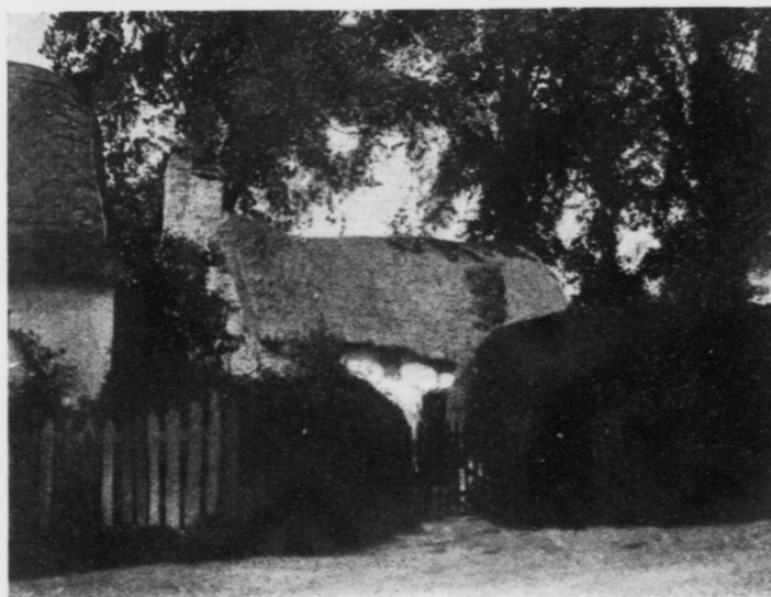
LABOURERS' COTTAGES AT COATE
