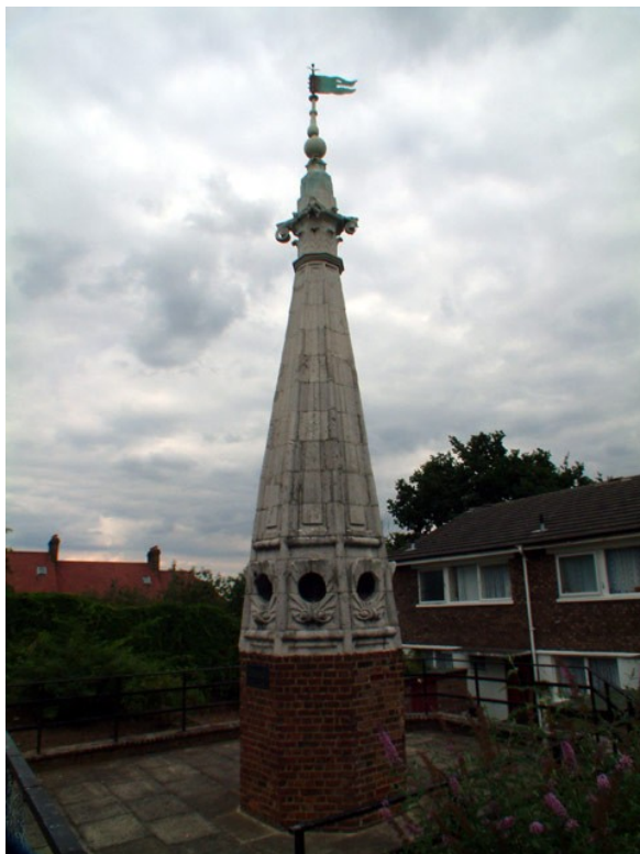
The apex of St. Antholin's church spire, mounted on a brick plinth, in Sydenham, SE26. It was statutorily listed in 1954.
